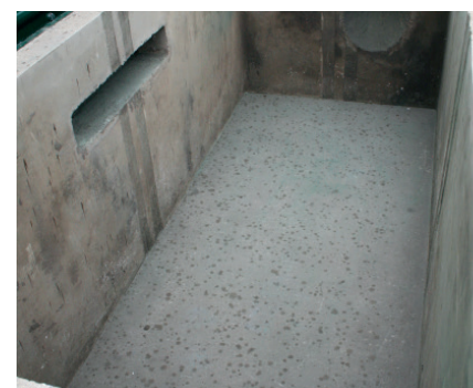
Internal Main Chamber View
