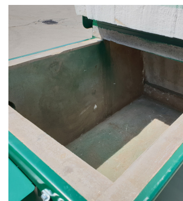
Internal Chamber View
