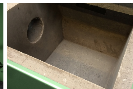
Internal Chamber View
